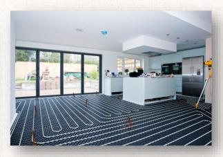
Underfloor heating is a heating system that embeds powerful and flexible tubing in the floor; heat radiated from the floor is transmitted to the walls, creating an ideal comfortable environment for that inside. It is both efficient and economical and has several advantages over radiators.
